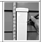
2. Align the screw holes in one of the saddle brackets from the rail kit with the horizontal line marked in step (1) making certain the bracket is centered on the wall plate. Mark the screw locations. Install the saddle bracket with the required screws as instructed in the rail kit.
